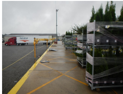
Concrete shipping and receiving pad.
